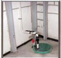
Sump Crotch & Wall Reinforcement
