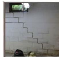
Wall Crack
