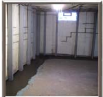
Drain Tile & Reinforcements
